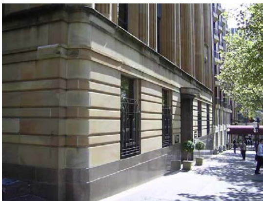
Street view of Transport House
